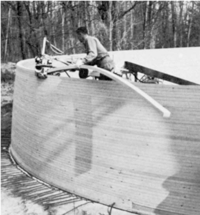
Figure 9.5 Dome-shaped buildings using PS foamed boards.
